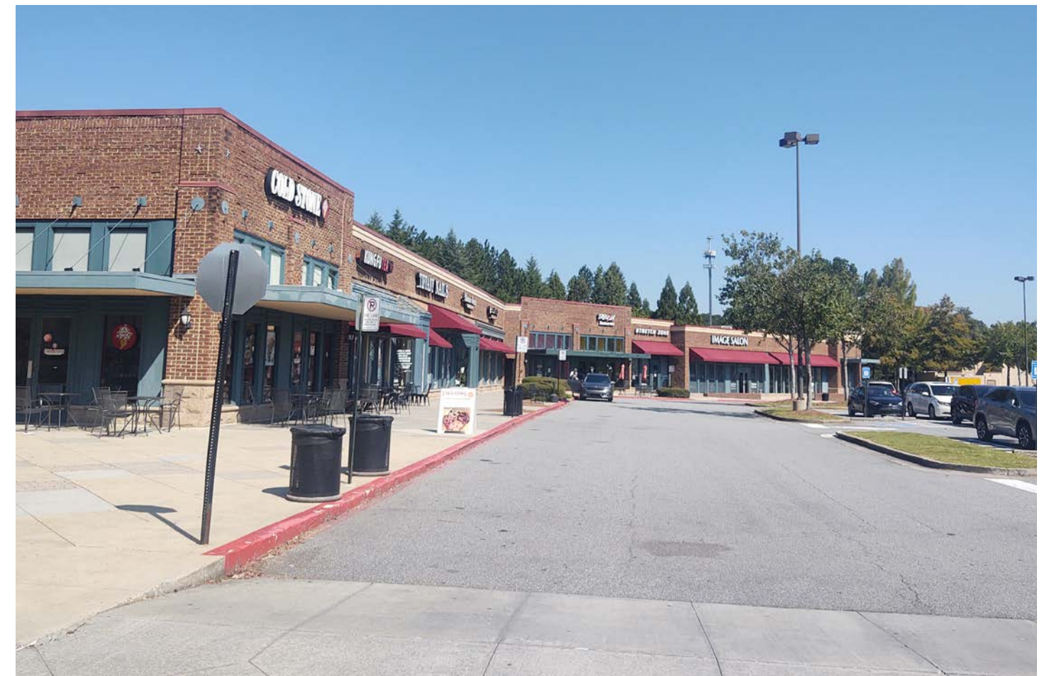
Image Caption: Existing retail on the development site at Regal Medlock Crossing
