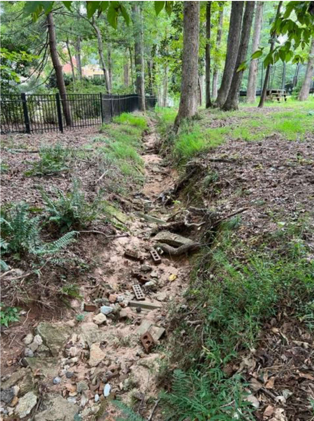
Dry Creek – Drainage Basin Behind The Liles Home
