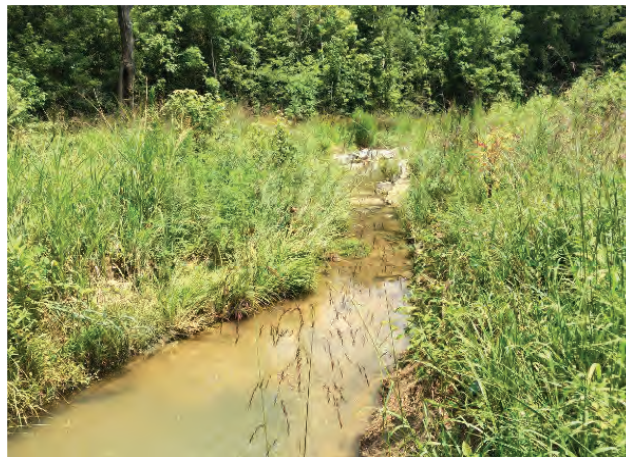
Photo 6 Completed Stream Restoration
